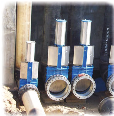
Mixing chamber installation
