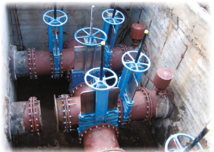
Sewage water treatment application
